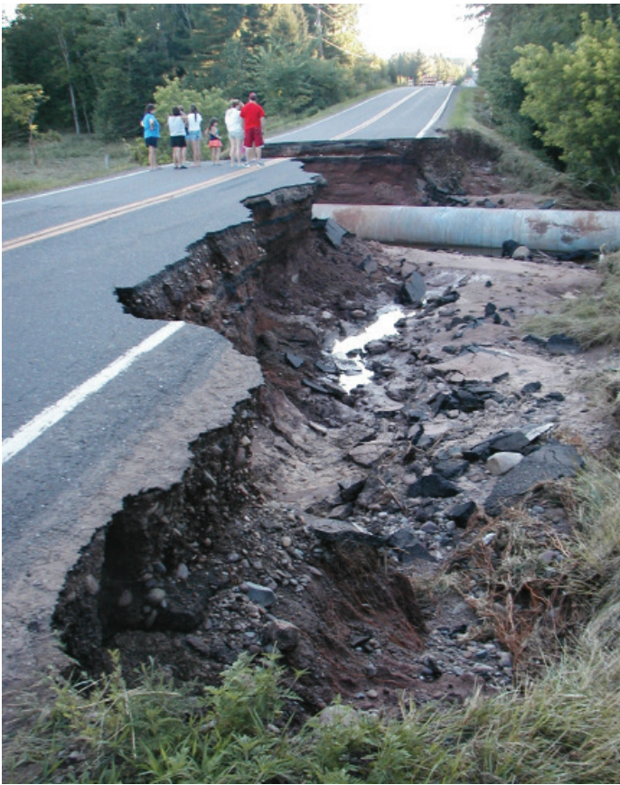
Culverts and other infrastructure downstream from areas with altered wetland hydrology receive more water, more quickly, making them more vulnerable to water-related damage.
